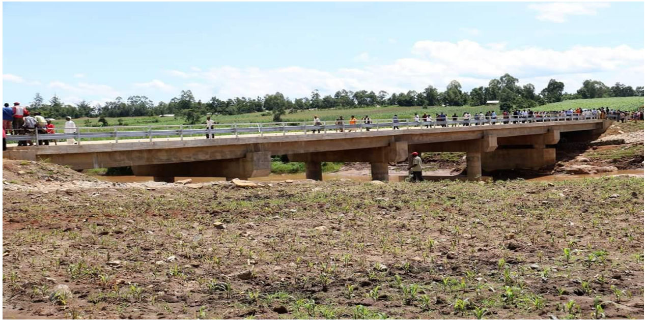
Photo 4: Khaunga Bridge constructed by the County government
