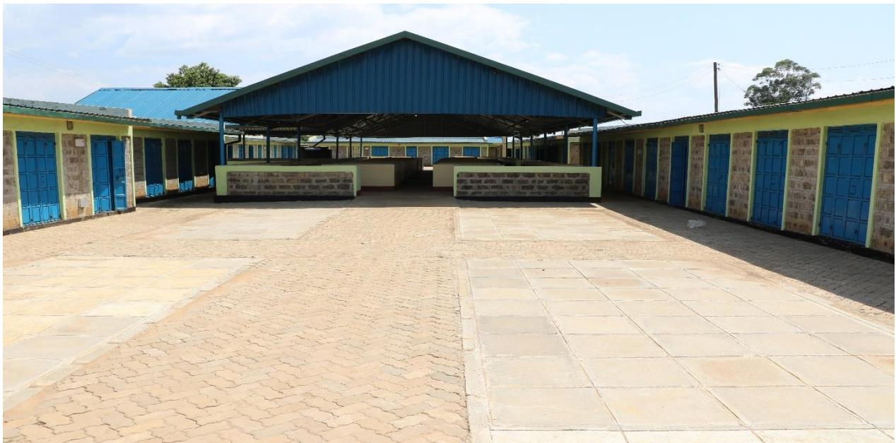
Photo 7: A market constructed by the County Government
